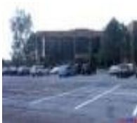
Building view,, we are located on the second floor: Suite 218
